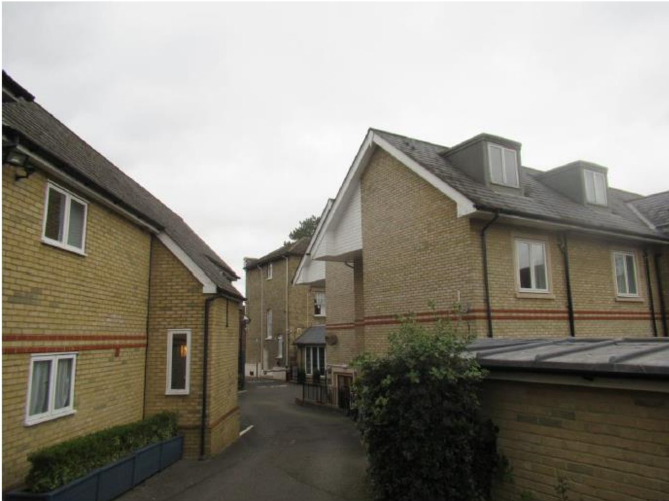
Access viewed from rear of site between the Hotel and the Coach House
